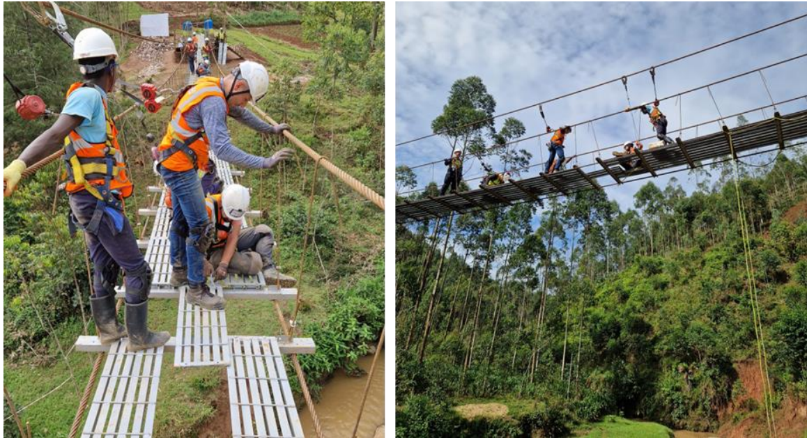
Figure 12 - Incremental installation of the deck
