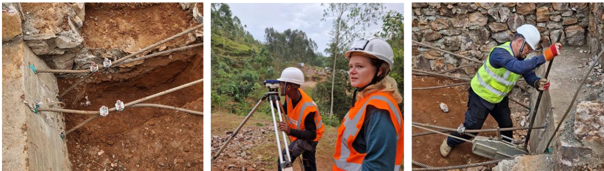
Figure 10 - Partial anchorage in the abutments and cable tension adjustment
