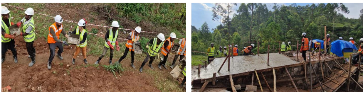
Figure 14 - Human chains for filling the abutments and concreting the access ramps
