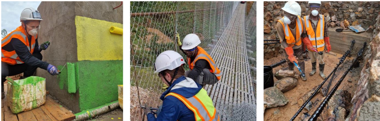
Figure 13 - Painting of the abutment towers, installation of fencing, and cable coating
