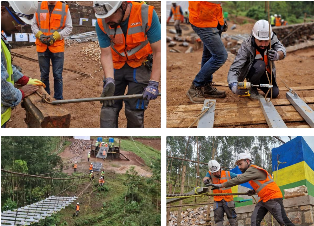
Figure 11 - Assembly and launching of the swings
