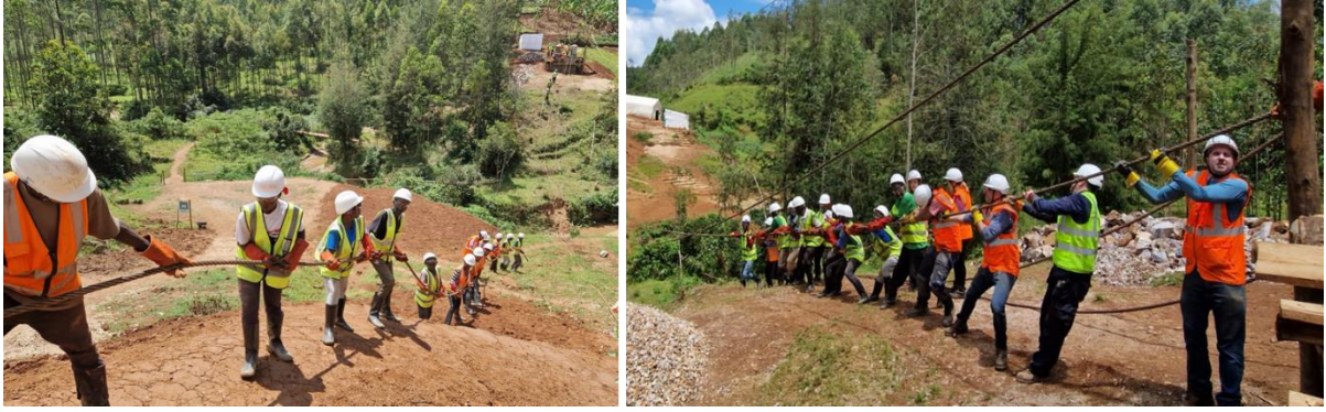
Figure 8 - Manual cable tensioning using arm strength
