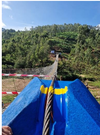
Figure 15 - Cable slip control marking
