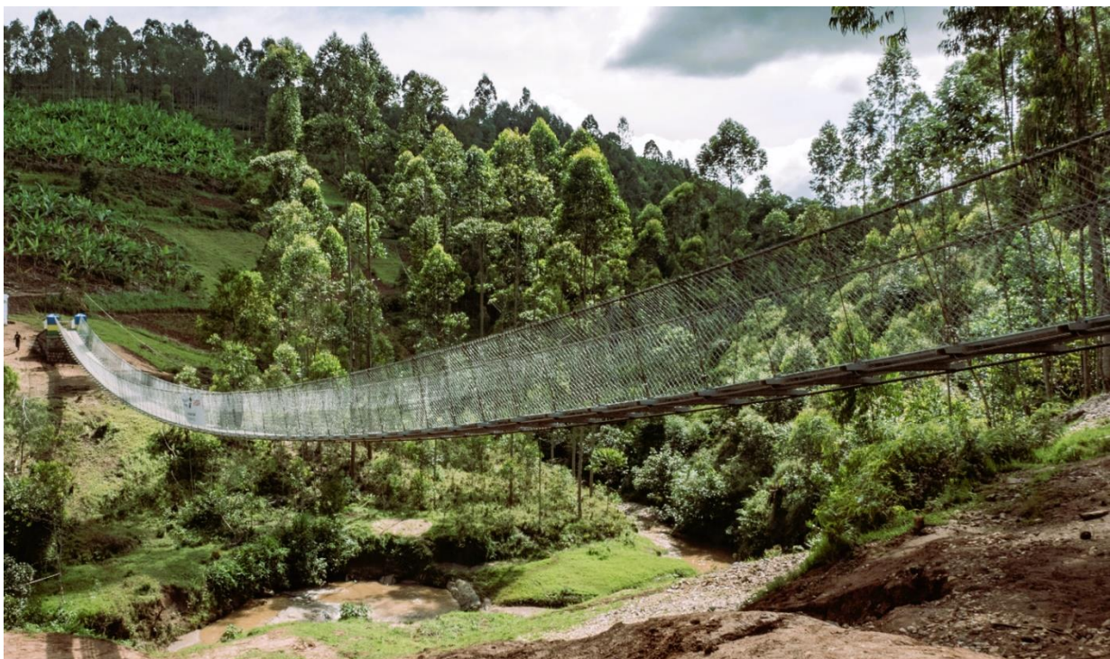
Figure 1 - The trail bridge over the Gikeri River in the Shyagari Valley
