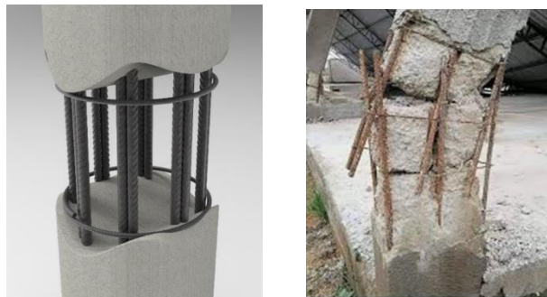
Image 8 – Overlap in a column (©BARTEC) and Overlap Failure (Internet)
