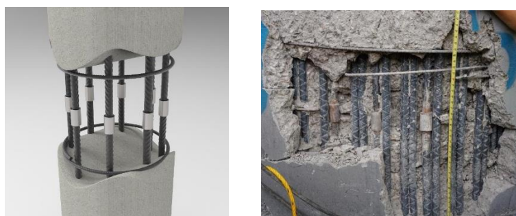
Image 9 – Mechanical splices in a column & Spliced rebars are not affected by the failure of surrounding concrete (2017 earthquake Mexico City – Internet)
